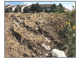
Soil erosion control
